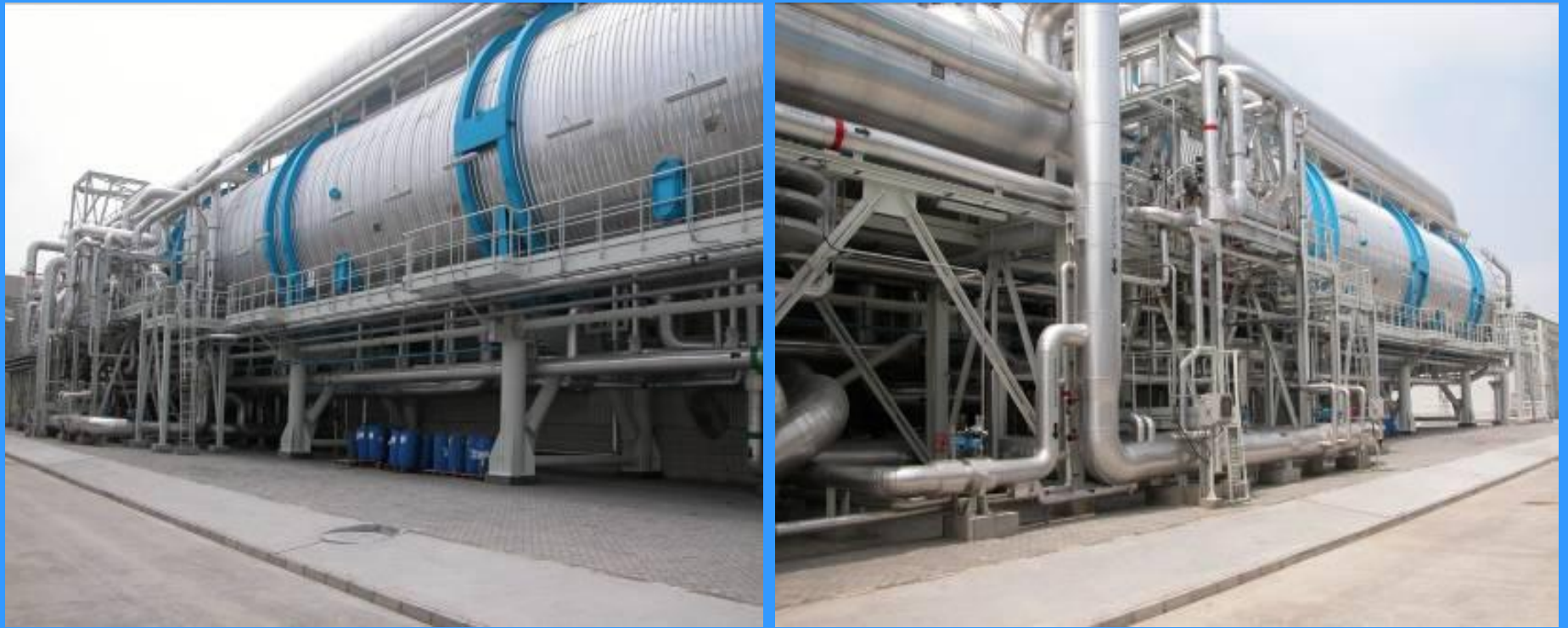
Fig.2-11 2 \times 10000 \text{ m}^3/\text{d} MED Equipments imported by Huanghua power plant in 2002
